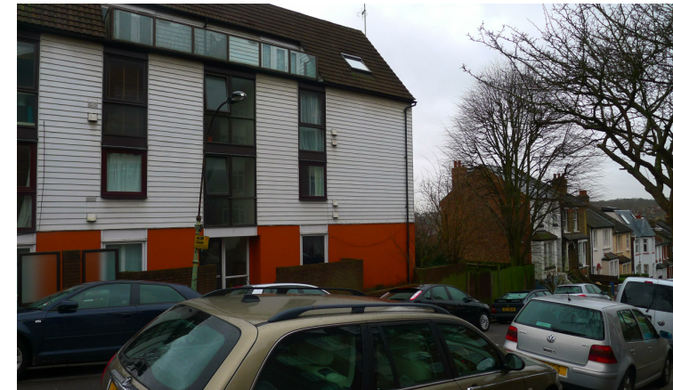
VIEW OF THE SITE AND ADJACENT BUILDINGS
