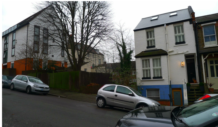
VIEW OF THE SITE AND ADJACENT BUILDINGS
